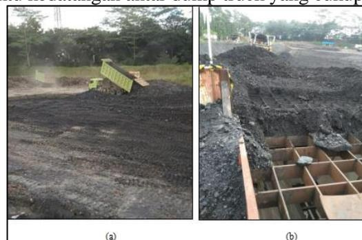
Gambar 15. Kegiatan (a) Dumping, (b) Trimming ke Hopper
