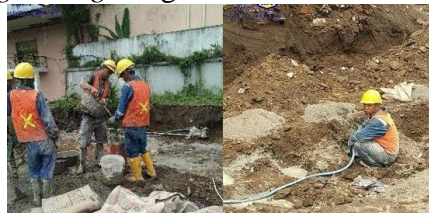
Gambar 5 Proses Grouting Soil Nailing
