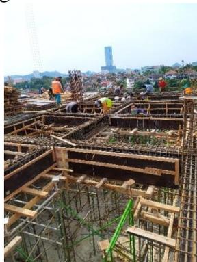
**Gambar 10 Proses Pemasangan Bekisting Balok**
